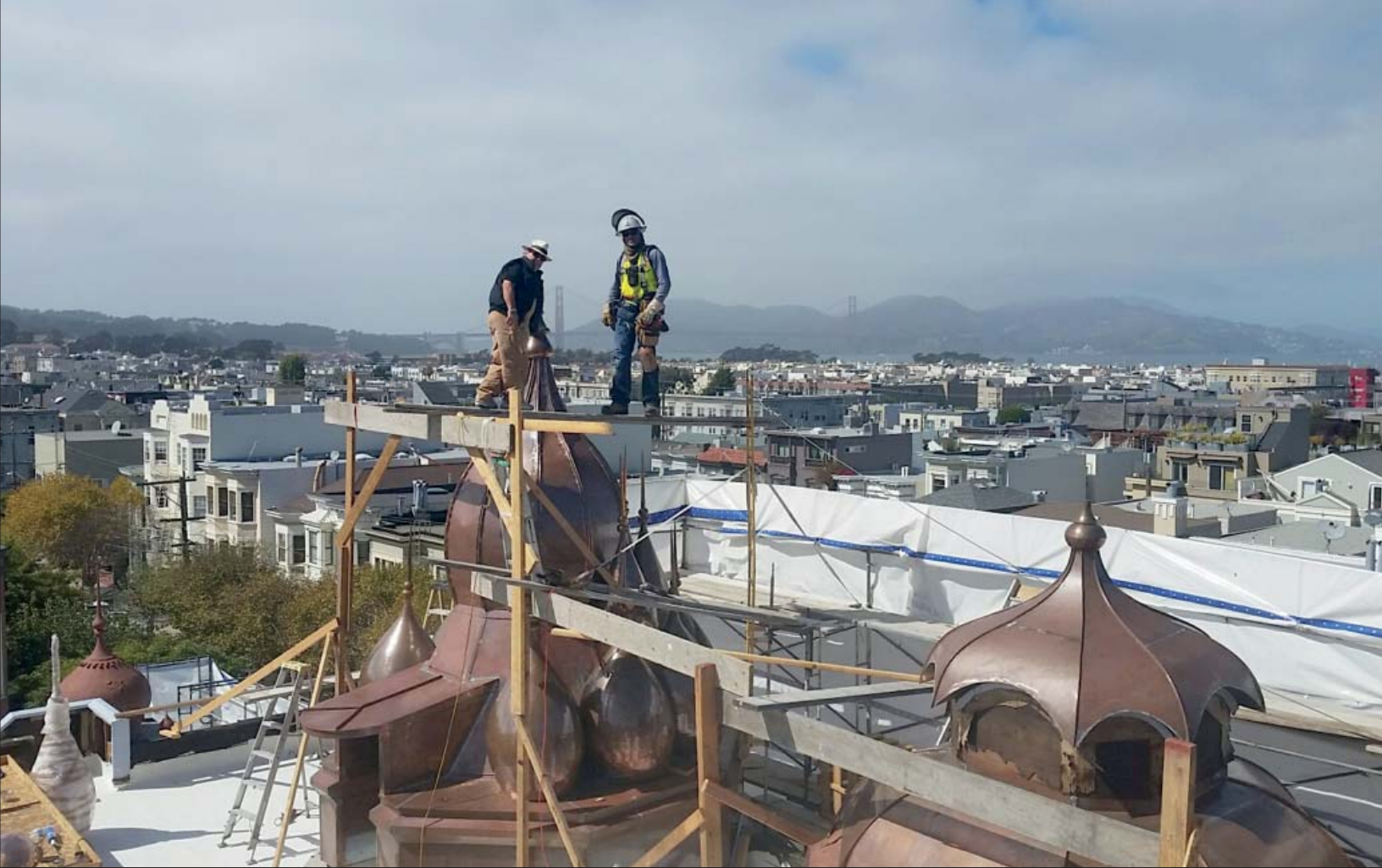
Scaffolding installation for tower work
