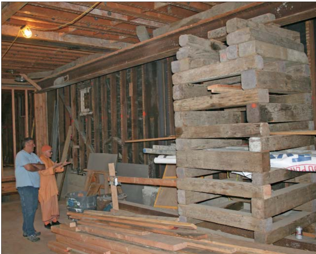
Steel beam support in the temple auditorium, December 2014
