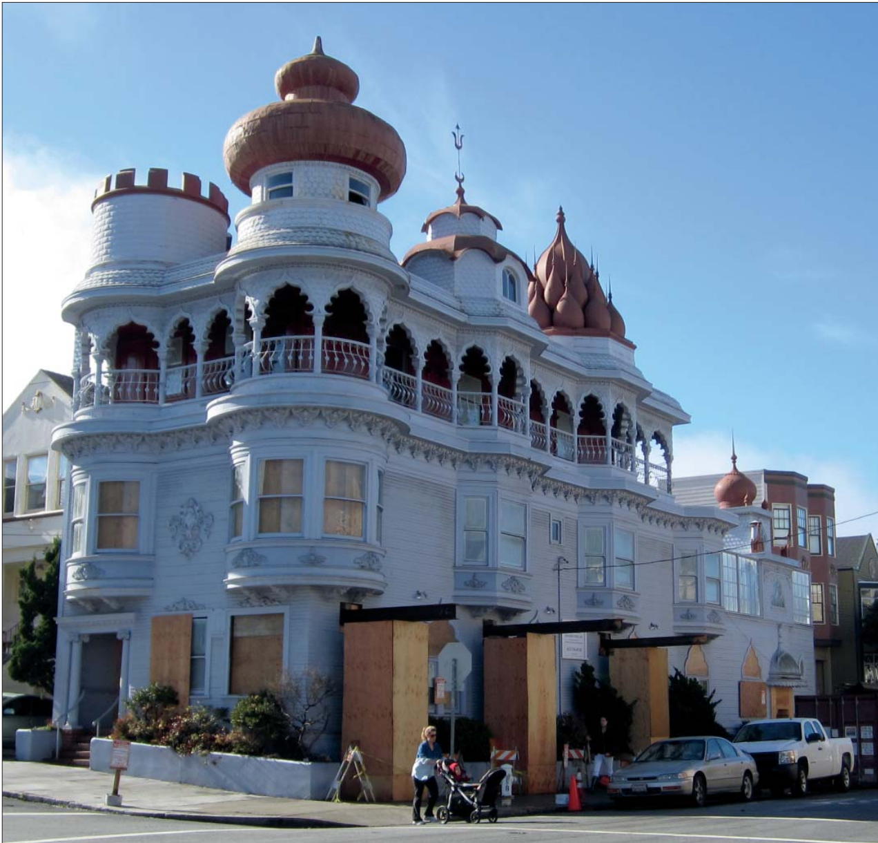
Old Temple temporary steel beam supports, November 2014
