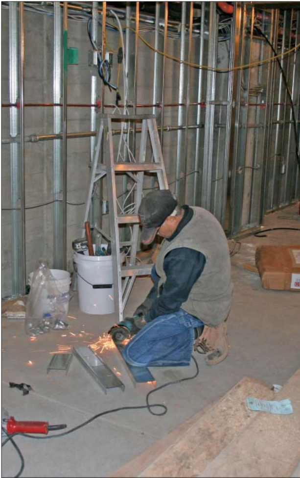
Cutting metal studs
