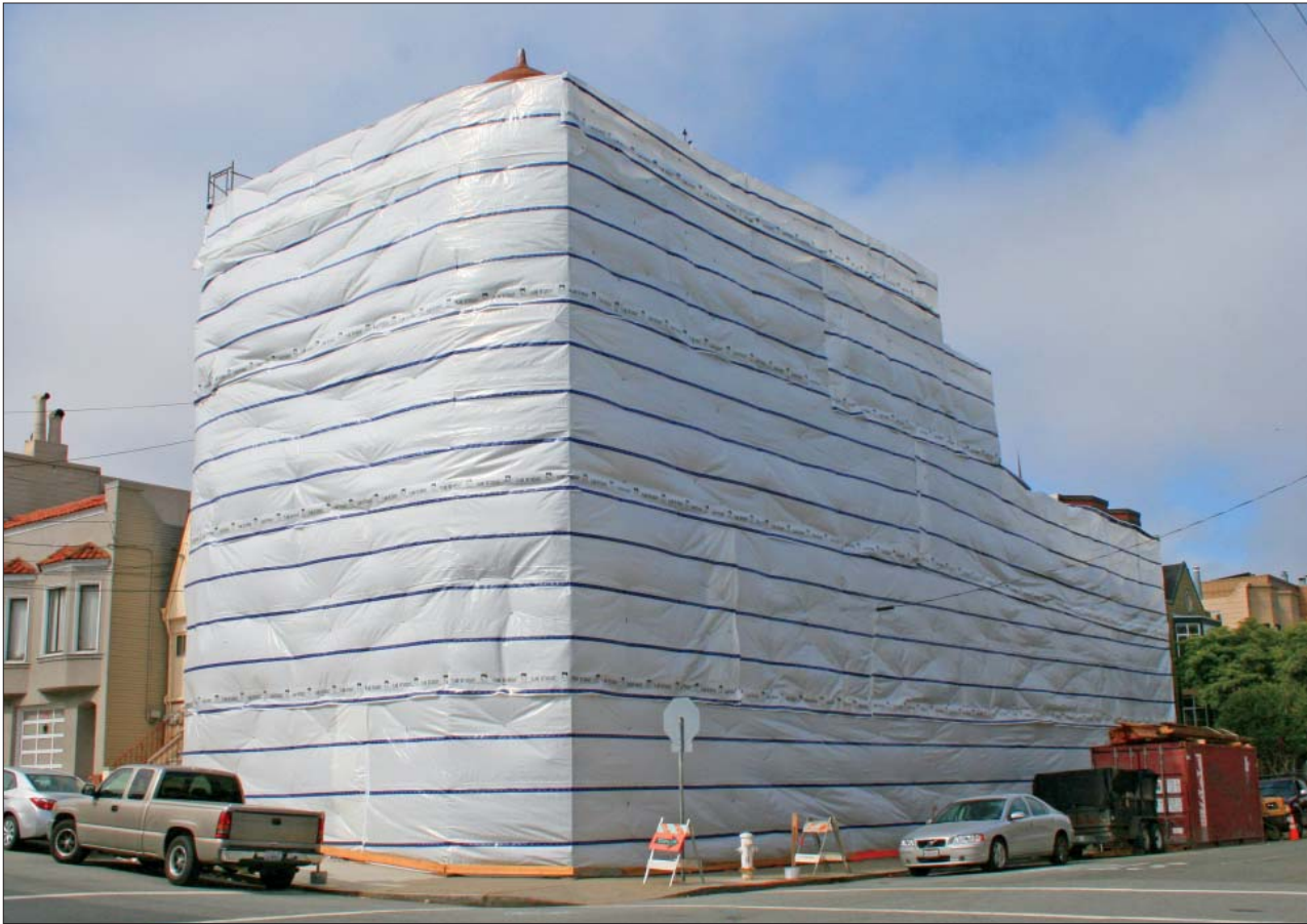
Protected by construction shrink wrap, May 2015
