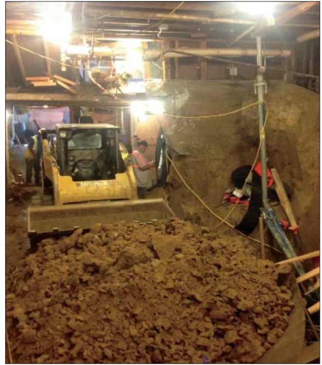
Excavation of basement, April 2015
