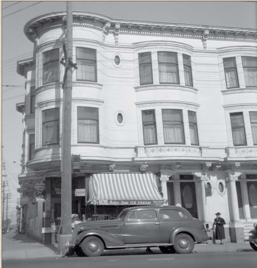
Above: 40 Steiner Street, top floor (1930s' photo)
