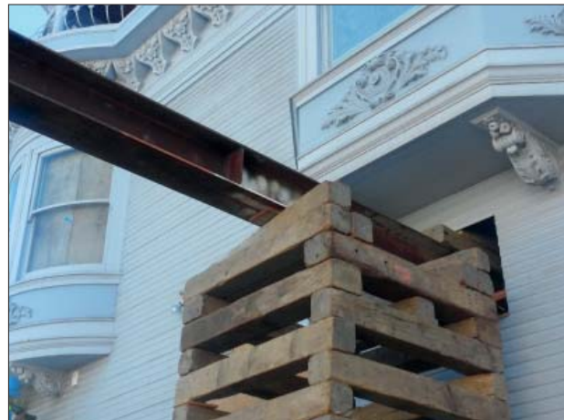
Closeup of steel beam support and cribbing
